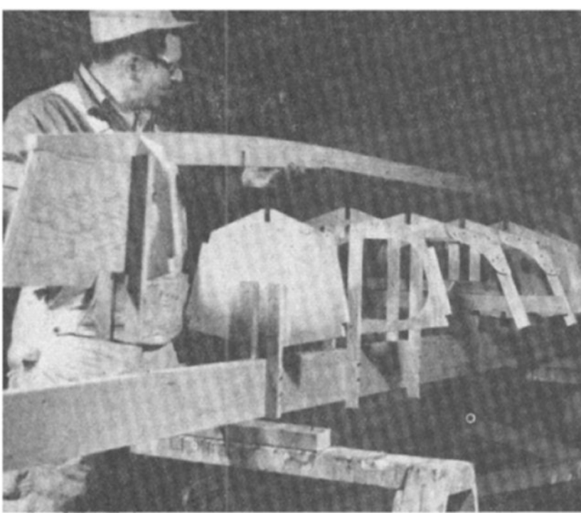
Fig. 1. All joints between keelson and frames should fit snugly. Remove keelson and daub glue in all frame joints. Replace keelson. Toe nail stem pieces to the center of the strongback.
