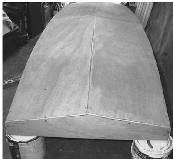
The exterior of this Cruising Mouse hull has been prepared for glassing the seams. The cable ties have been cut off flush, and the edges have been gently rounded with a rasp. (Anthony Smith)
