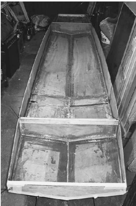
A stitch-and-glue Cruising Mouse hull made by Anthony Smith is nearly complete. The seams between all the hull panels and bulkheads have been filleted with epoxy-based putty and taped over with fiberglass tape and more epoxy. (Anthony Smith)
