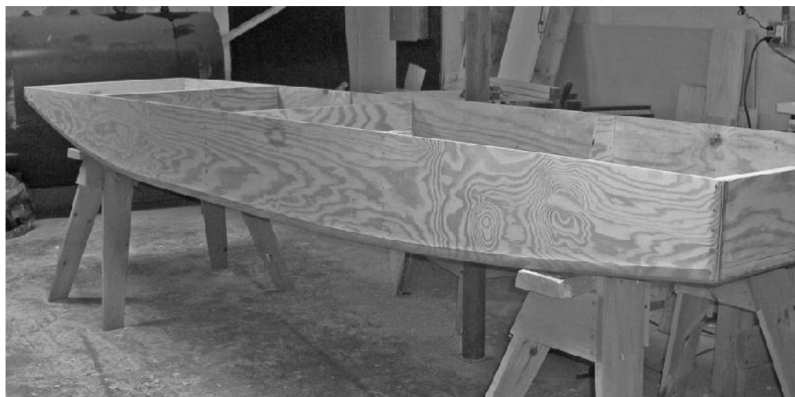
A Lilypad hull with transoms, bulkheads, and open-topped frame in place. The builder combined aspects of two construction methods, using the more carpentry-intensive simplified chine log method for bulkheads, frame, and transoms, and the stitch-and-glue method for the long side-to-bottom seams. (The outside seams have been taped; the inside seams have yet to be filleted and taped.) (Robert Holtzman)
