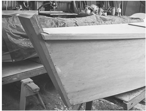
FIGURE 7-12. An outer stem is glued in place and shaped round and fair with the hull panels.
