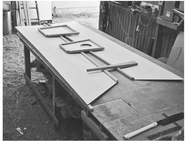
FIGURE 7-9. Bulkheads, side panels, and stem ready for assembly.
