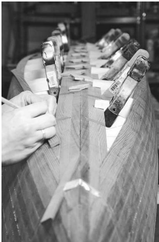
Figure 6-34. This kayak is being stripped up using the side herringbone pattern using book-matched strips without staples. It takes a lot of U-jigs clamped in place to hold the strips as the hot-melt glue cools. A stubborn strip on the left side is being held down with some tape.
