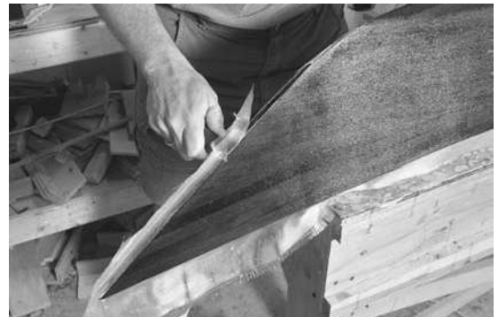
Figure 13-46. After the epoxy has begun to cure, you can trim off excess glass. It is best to do this trimming while the epoxy is still green, or a little soft. How soon after applying the resin this is depends on the epoxy you are using and the temperature in your shop. I usually check a couple of hours after finishing the fiberglassing.
