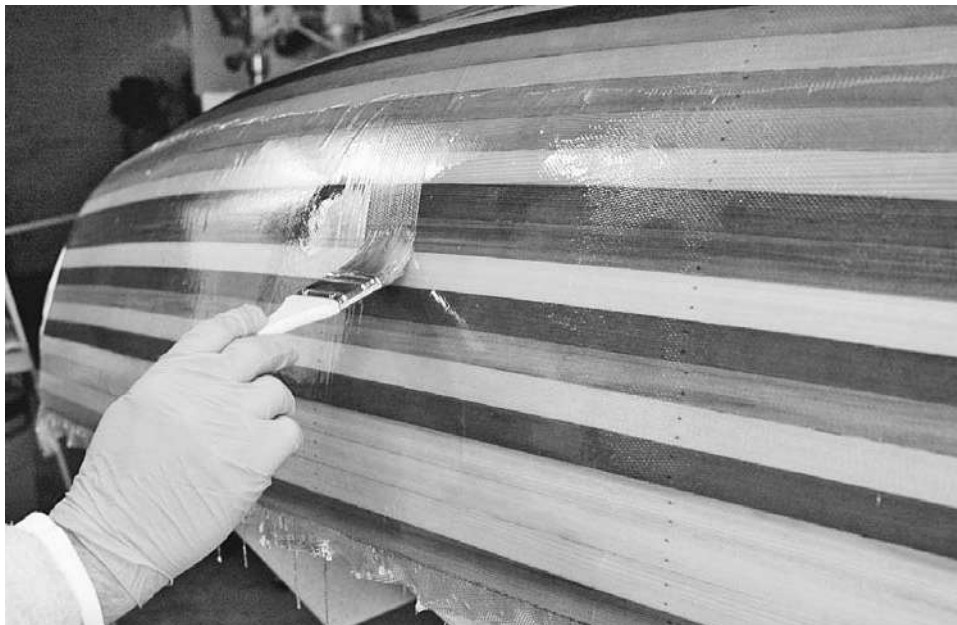
Figure 11-20. The fill coat fills up the fabric texture (right) to create a smooth finish (left). Brush on the epoxy using the same crisscross technique you will eventually use to apply varnish.
