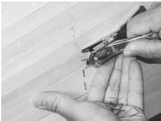
Figure 6-42. A heavy-duty office staple remover makes quick work of pulling the staples. I've filed down the blade a bit to make it easier to shove under the staple, but it easily lifts the staple with minimum damage to the wood.
