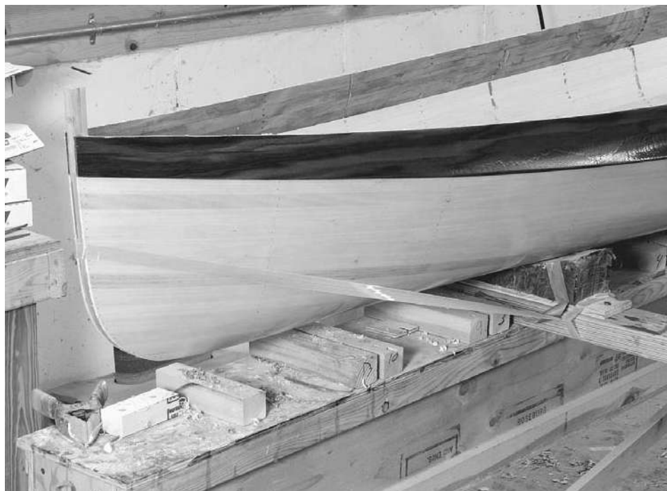
Figure 7-19. The boat will be very light when you remove it from the forms and start working on the inside. Strategic use of strapping tape keeps it from wandering around as you clean up the interior.
