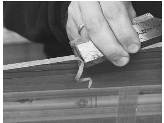
Figure 13-41. After using a saw to rough out the cockpit area, trim it to fit the recess assembly using chisels, planes, rasps, and/or sandpaper. Start with the hole a little undersized and work around the edges until a tight fit is created.
