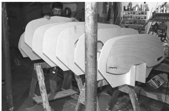
Figure 5-18. The slotted strongback is very simple to set up. Two long beams with slots cut in them accept matching slots on the forms. Drop the forms into the slots, make sure they are seated all the way down, and you are good to go.
