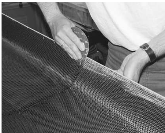
Figure 9-31. Before joining the deck and hull, rough up the epoxy and fabric along the edge to assure a strong bond.
