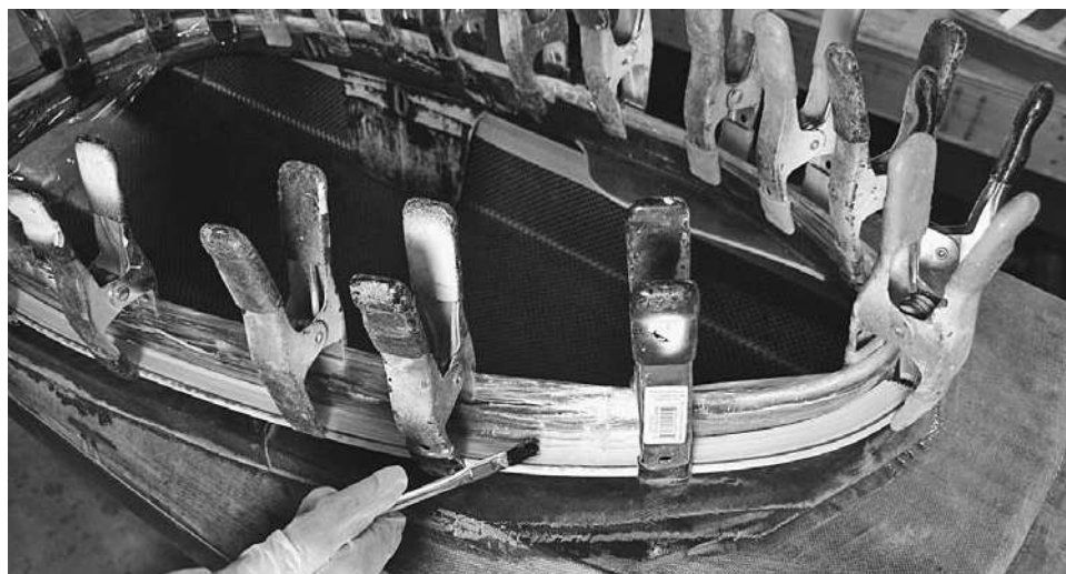
Figure 13-53. I usually finish the coaming at this time, but you could do these steps anytime after installing the riser. I use the coaming riser as a form to laminate the coaming lip. The strips should be about \frac{3}{16} to \frac{1}{4} inch wide and about \frac{1}{16} to \frac{1}{8} inch thick to make the bends. You will need enough strips to make a lip \frac{3}{4} to 1 inch wide. Wrap the coaming riser with tape or stretch wrap (either plastic food wrap or binding wrap available at office supply or woodworking stores) so the laminations do not end up glued in place yet. The strip length should be just short of long enough to go all the way around the cockpit.
