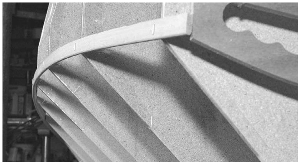
Figure 11-12. Get your eye down near the first strip to make sure it runs in a smooth, fair curve. If you see a wiggle, pull out the staple and let the strip bend naturally. Check to see if the curve is now fair. If it is, just run a staple into the strip where it is without moving the strip. If the curve is not yet fair, try removing some more staples. If this does not work it is probably because the strip itself has a kink in it. You could just pop it off and try another strip or try restapling the strip so it is fair.
